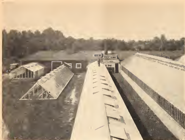
General greenhouse range. Narrow house for propagation. Small houses for quarantine.
